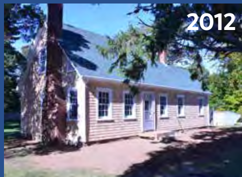
2012 Littlefield House Renovation
