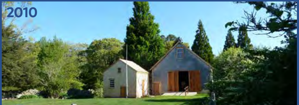
2010 Far Barn Renovation
