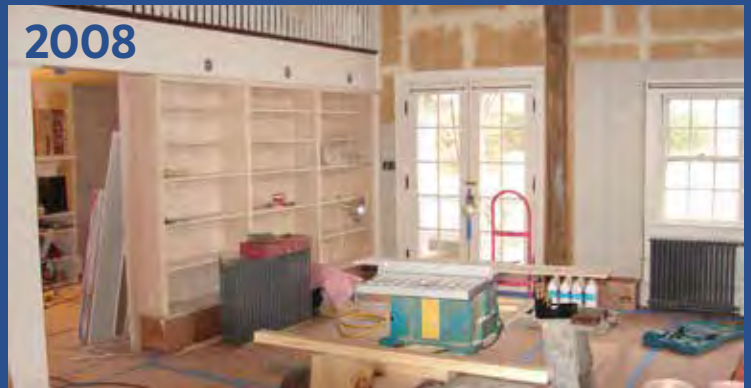
2008 Cow Barn Renovation
