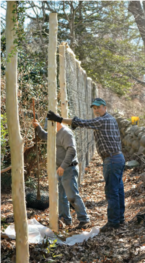
Tucker helps with fence construction during the renovation of Polly's Playpen.
