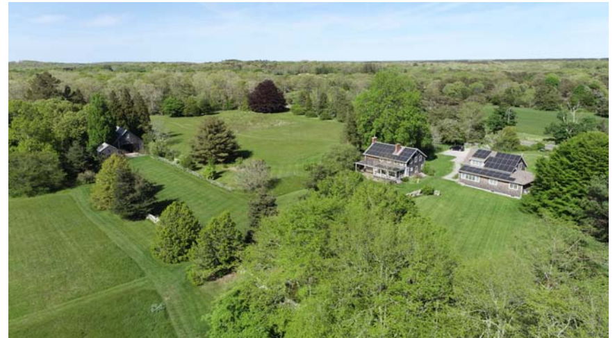
Figure 2 The new houses will harmonize with the Arboretum's historic buildings and landscape.
