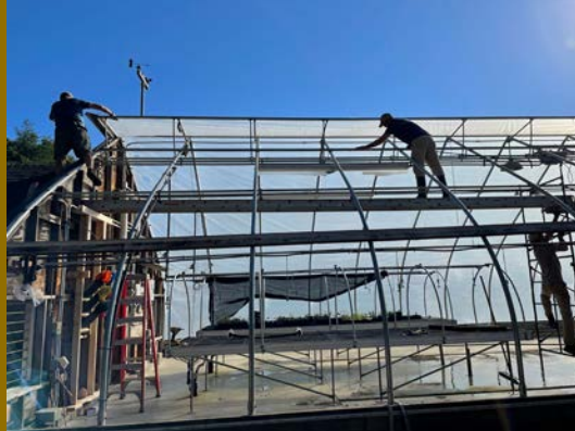
Staff replace plastic on one of the PHA greenhouses.
