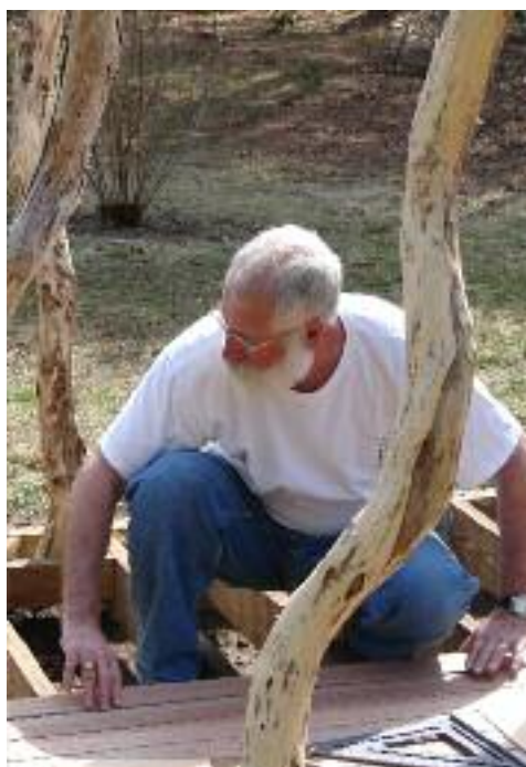
Gary Montrowl works on the Bower project.
