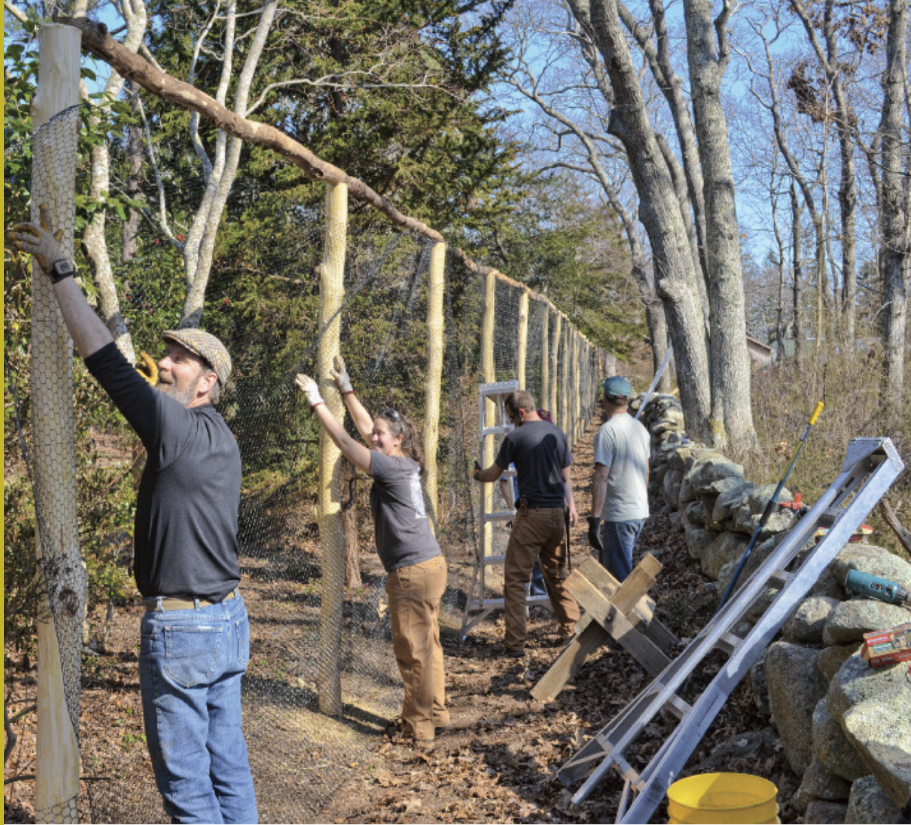
The Playpen renovation project is another example of preservation at the PHA.
