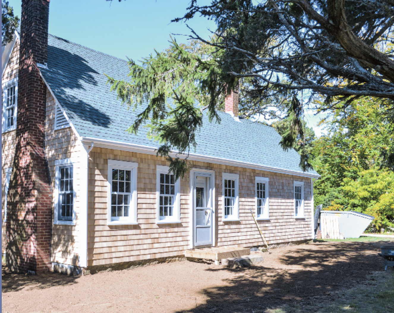
The Littlefield House renovation project
